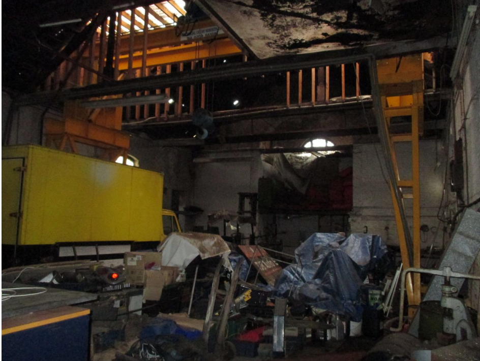
Ground floor Mission Hall building, looking west:
